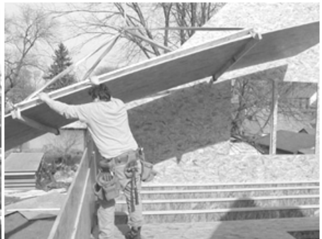
Fig. 3 Placing OSB panel floor between wall panels
