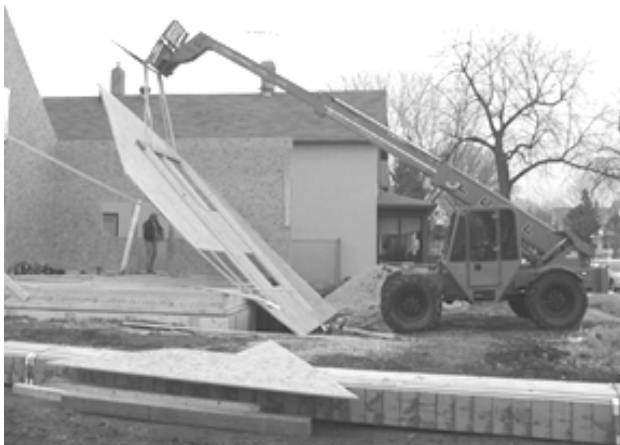
Fig. 2 Pilot House (House One) Lifting the gable end wall
