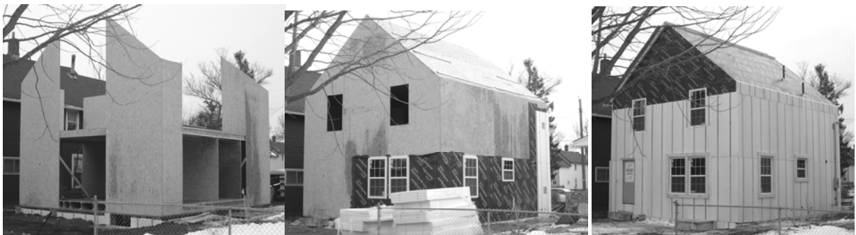
Fig. 5 House Three first panels w/ 4x4 corners panel shell w/ partial membrane insulation over wall and roof membrane
